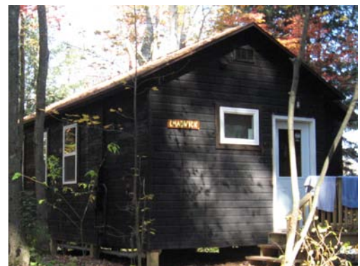
Chadwick was fully renovated and expanded.
